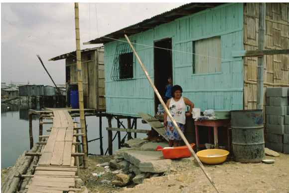
13. Informal home and toilet/bathhouse built over the water in Ecuador. Santiago de Guayaquil, Ecuador, 1999.
