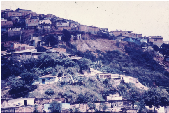
9. Dense informal settlement built up hillside. Note the high risk for landslide of many structures. Caracas, Venezuela, 1989-1995.
